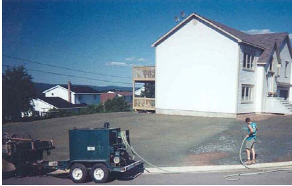
Figure 5-1. One-step Hydraulic Seeder at an NBHTA Topsoil Conservation Project.
